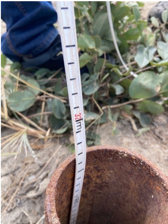
Figure 13 Depth of boreholes lying partially fallow in the bush and drilling near Shamangorwa. (©MUDIRO/2021/BMueller)
